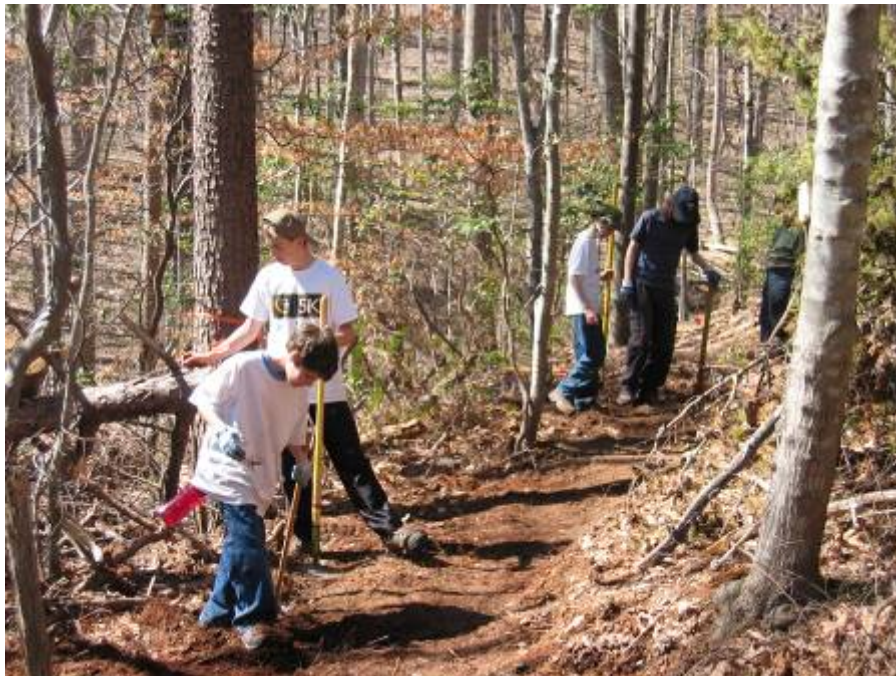
The Scouts at work making a “bench” cut.
